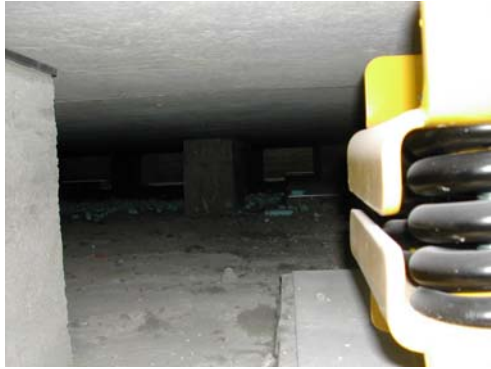
Figure 5. The elastic suspensions of the whole system
