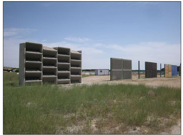
Figure 4. Overview of the Valladolid test site. From left to right: non flat absorbing green wall, non flat absorbing porous concrete A3, non flat absorbing porous concrete A2, flat absorbing timber barrier, Flat absorbing wall, strongly non flat metallic wall (the latter is the same sample in Figure 1).
