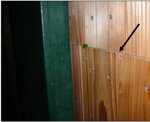
Fig. 17—The measurement junction between the timber boards on the rear side of timber/metal panels. The acoustic leak is indicated by the arrow (Picture taken during night time measurements).
